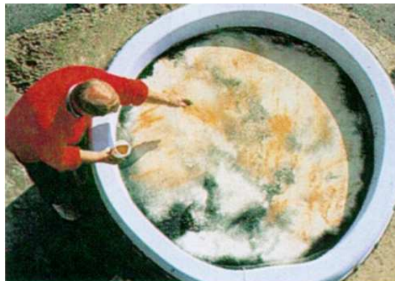
Dosing the MICROCAT-XRT over the oil layer.
